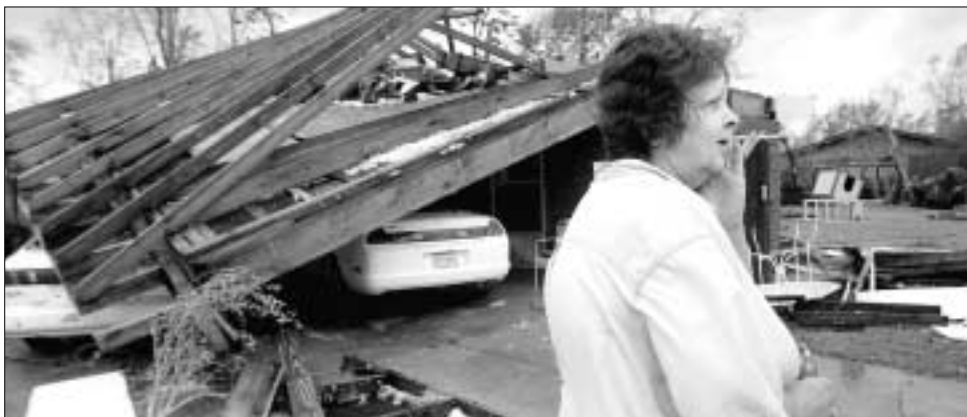
Cathy Breazeale of Gulfport, Miss., surveys damage to her home caused by Hurricane Katrina Aug. 29.
